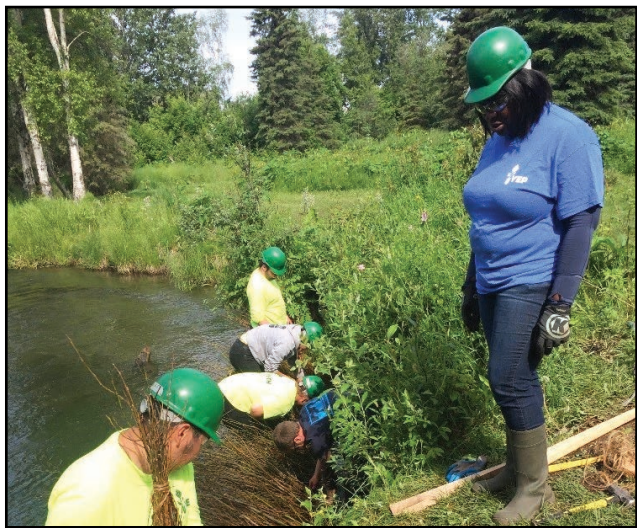
Anchorage Youth Employment in Parks crew restore 1,200 feet of Campbell Creek at Lynnwood Park in Anchorage. They used coir logs, brush layering, vegetative mats, live willow stakes, and plantings of native trees and shrubs to stabilize the streambank.
