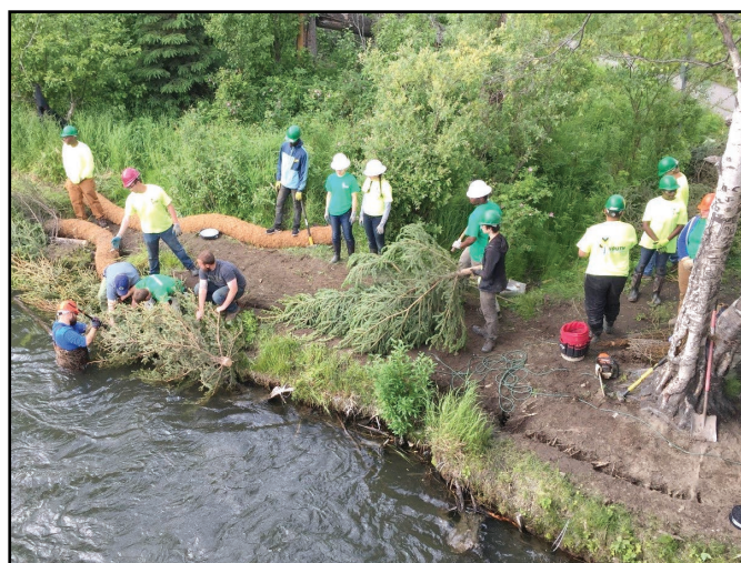
Anchorage Youth Employment in Parks crew stabilizes and restores banks of Campbell Creek in Anchorage. The crew also installed 50 feet of elevated, light-penetrating boardwalk for fishing access. Photo by Stephen Nickel
